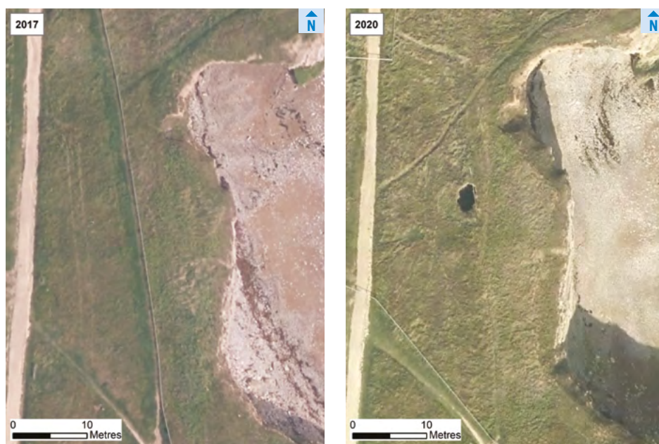
Figure 10. Opening of a 'sink hole' in the cliff top at Whitburn Coastal Park in South Tyneside, between 2017 (left) and 2019/20 (right).
