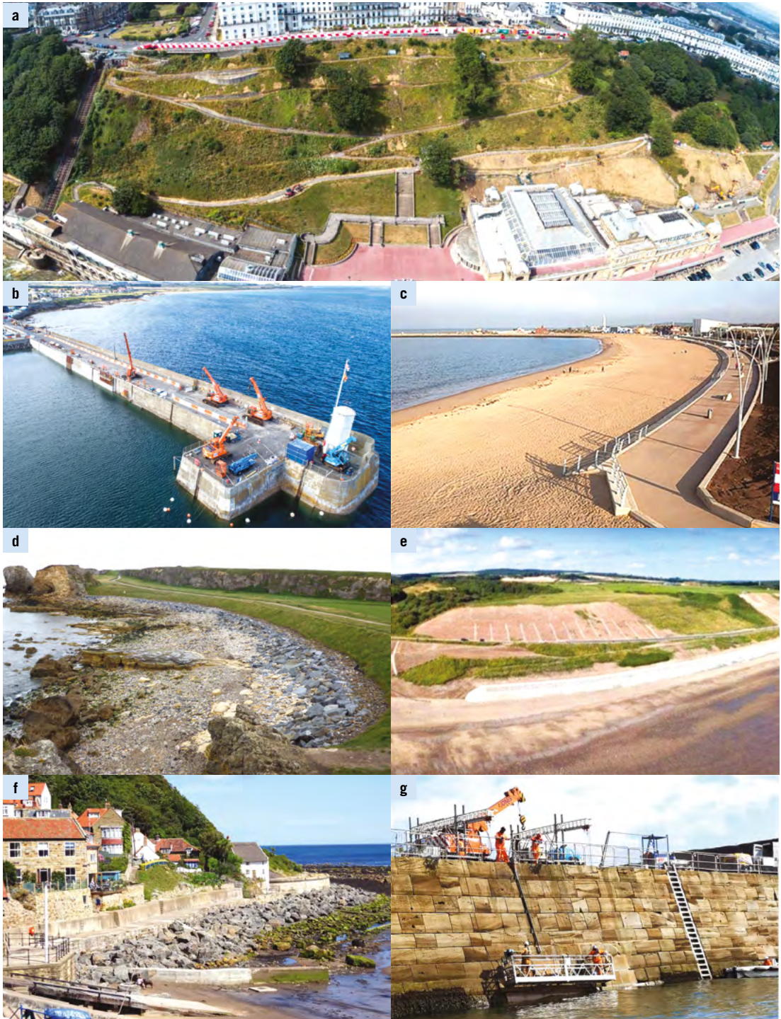
Figure 3. Coastal defences within Cell 1:
